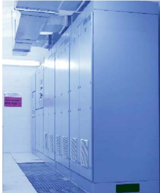
One of the two rows of cabinets including a connection unit, a voltage converter and control electronics in addition to the capacitors
