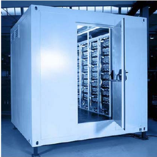
A SITRAS ® SES unit can absorb the braking energy released by all stopping trains within a radius of up to three kilometres (almost 2 miles)
